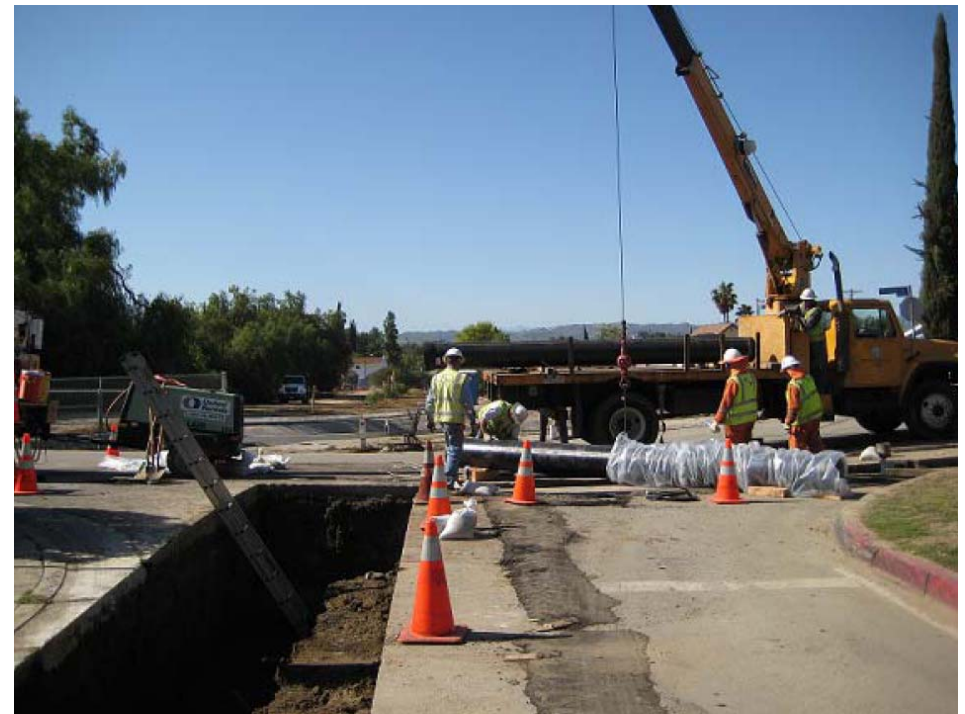
MULHOLLAND PIPELINE Project - 30065 (MARCH 2010)
